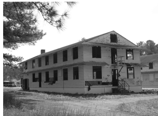
PHOTOGRAPH 1. Typical case study building at Ft. McClellan Army Base
