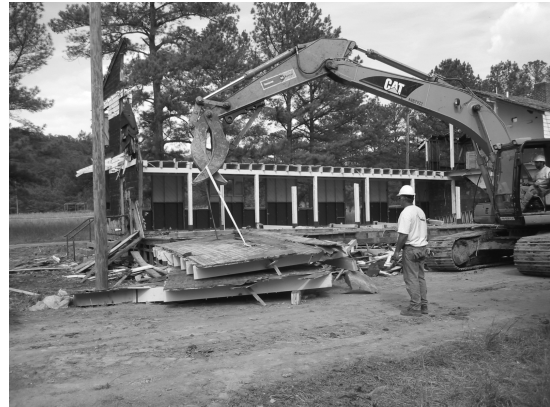
PHOTOGRAPH 3. Second floor panelization and lay-down for hand disassembly
