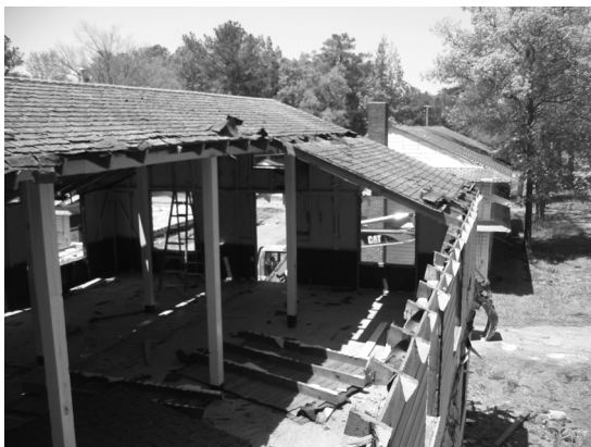
PHOTOGRAPH 2. Roof panelization
