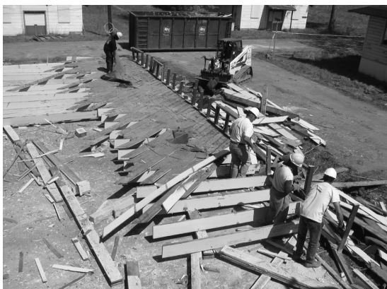
PHOTOGRAPH 5. Hand disassembly of dropped second floor
